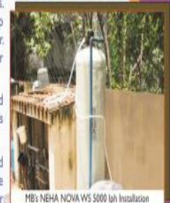
MB's NEHA NOVA WS 5000 lph Installation
