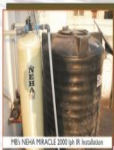
MB's NEHA MIRACLE 2000 lph IR Installation
